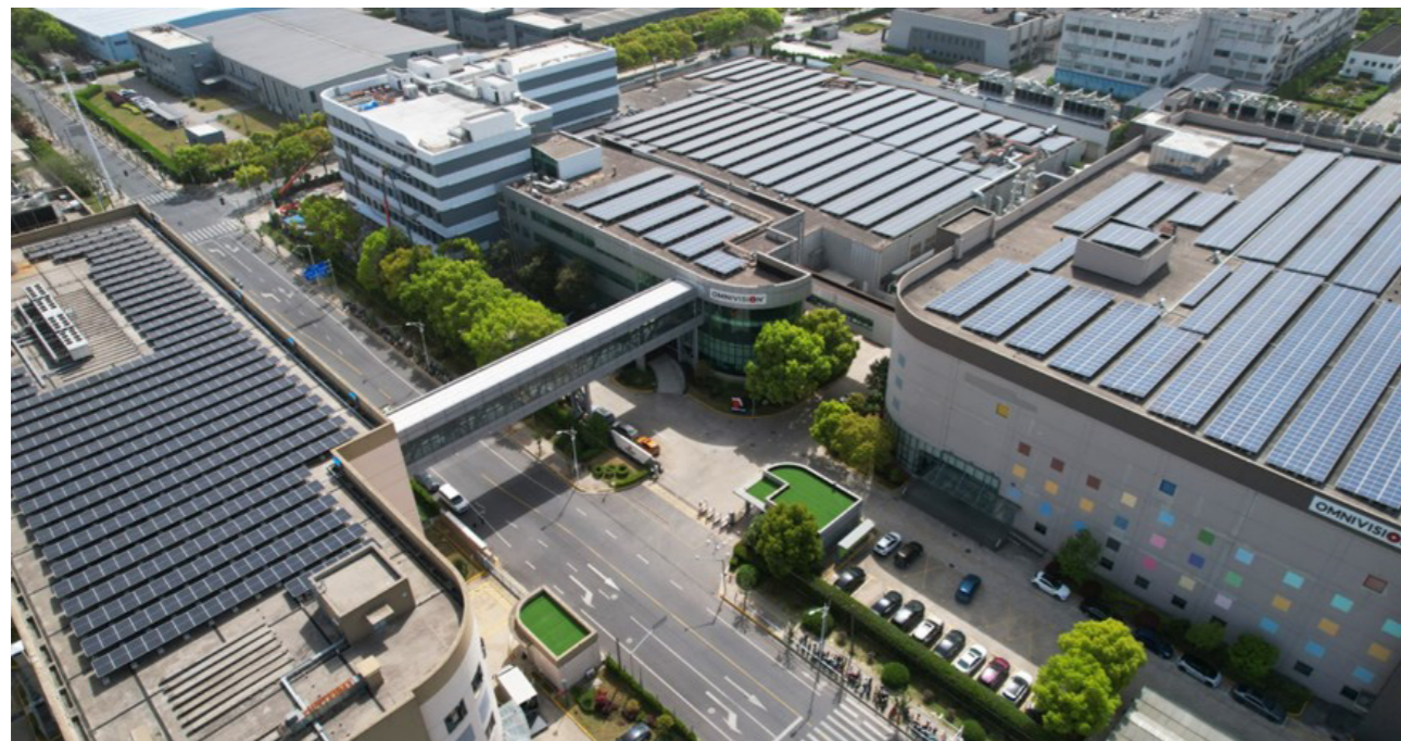
▲ Rooftop photovoltaic power generation at Shanghai Songjiang Park
