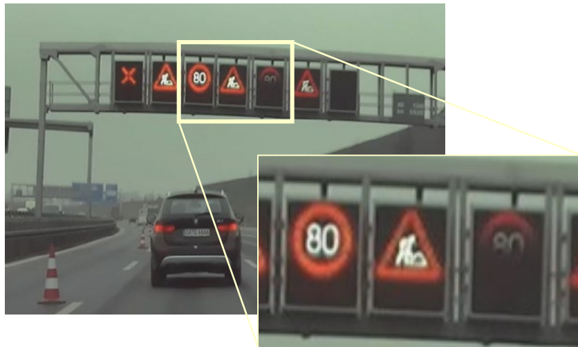
Figure 1. LED image flicker can create a problem in HDR camera systems for traffic lights, as shown in the close-up.
